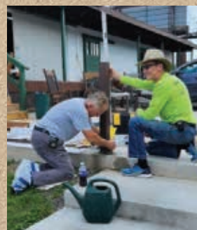
Sam and brother-in-law Jim, installing the railing... days before the wedding.
