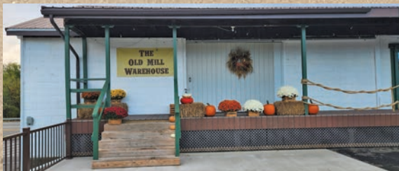
October 2025 - Ready for the grand reopening of The Old Mill Warehouse that took place October 18, 2025
