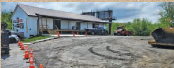
Renovations included paving the parking lot in front of The Old Mill Warehouse.
