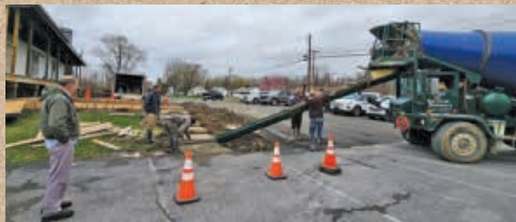
New concrete steps added for easier accessibility to the Old Mill Warehouse from the store parking lot
